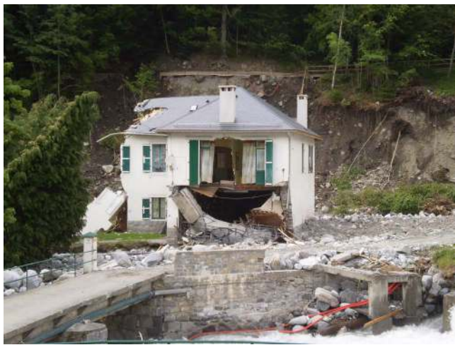
Fig. 1. House destroyed by the Bastan flood on the 18th of June 2013 in Barèges, in the Hautes-Pyrénées (photo taken on the 03/07/2013, S. Carladous).
