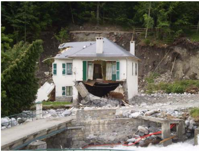
Fig. 1. House destroyed by the Bastan flood on the 18th of June 2013 in Barèges, in the Hautes-Pyrénées (photo taken on the 03/07/2013, S. Carladous).
